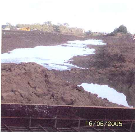
Open Channel 1500 meters long
