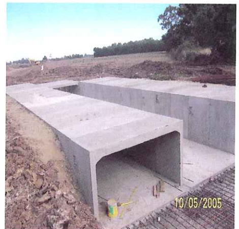
Box culverts installed prior to cover slab
