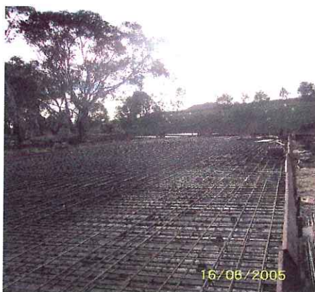
Heavily reinforced cover slab
