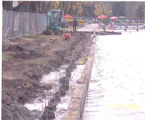
Sheet Pile Wall
