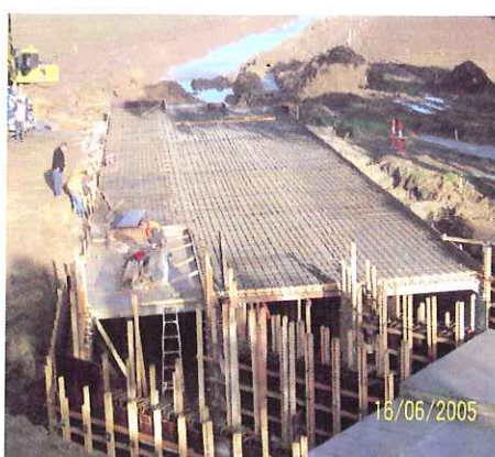
Insitu transition structure between culverts
