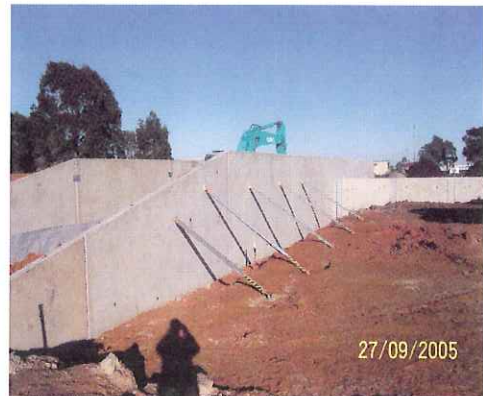
Tilt slab push pits.
