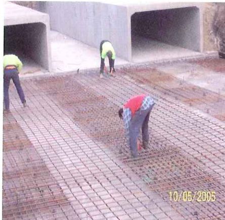
Steel fixing for culvert slabs
