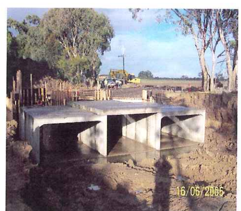
Upstream of Culvert
