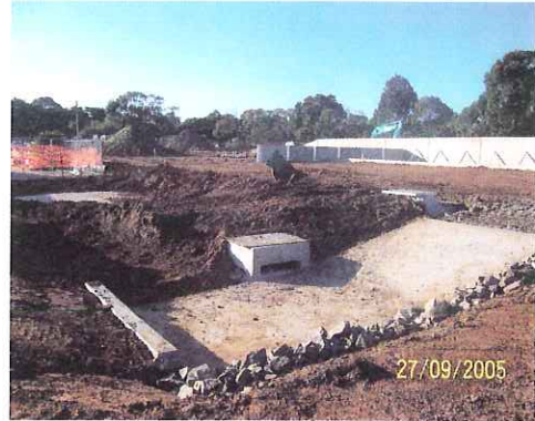
Wetlands Area looking back towards new push pits.
